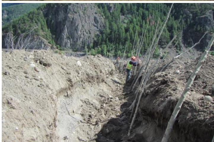
Figure 29 Live stake cuttings at the Gun Creek Fan east side, planting with a combination of machine and manual labour.
