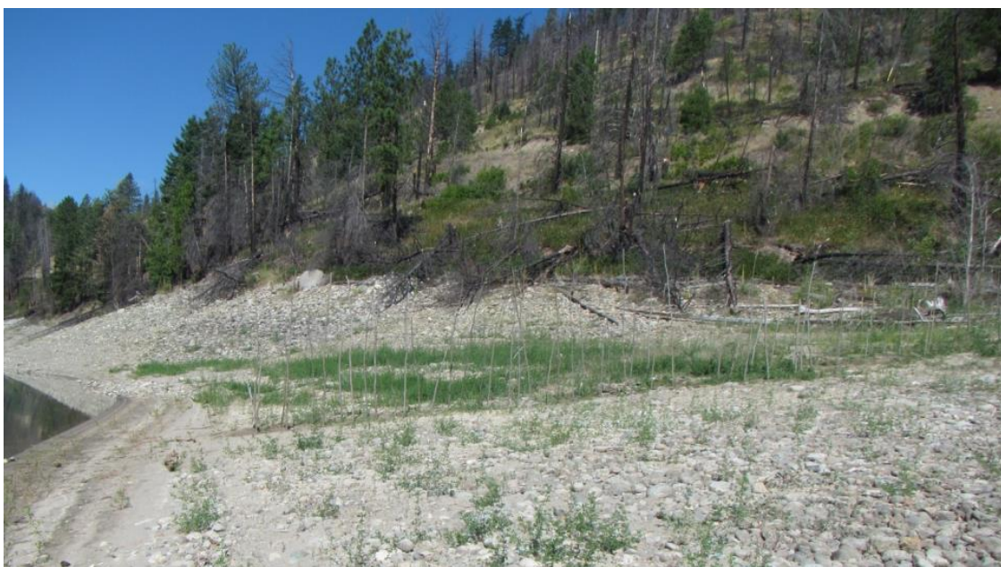
Figure 23 Live stake cuttings at the West end of the steep beach polygon STB02.
