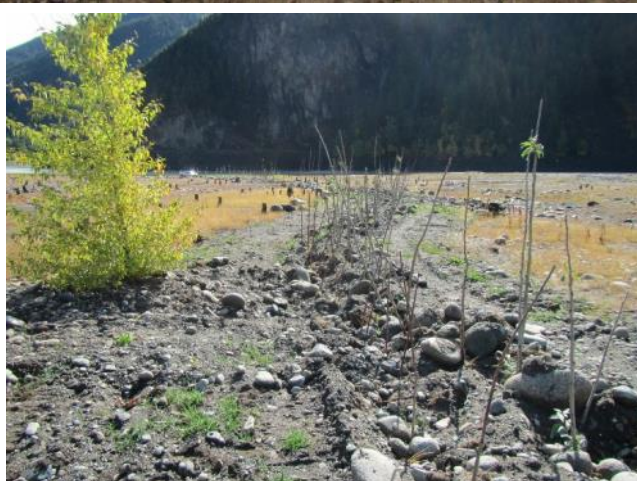
Figure 29 Live stake cuttings at the Gun Creek Fan east side, planting with a combination of machine and manual labour.
