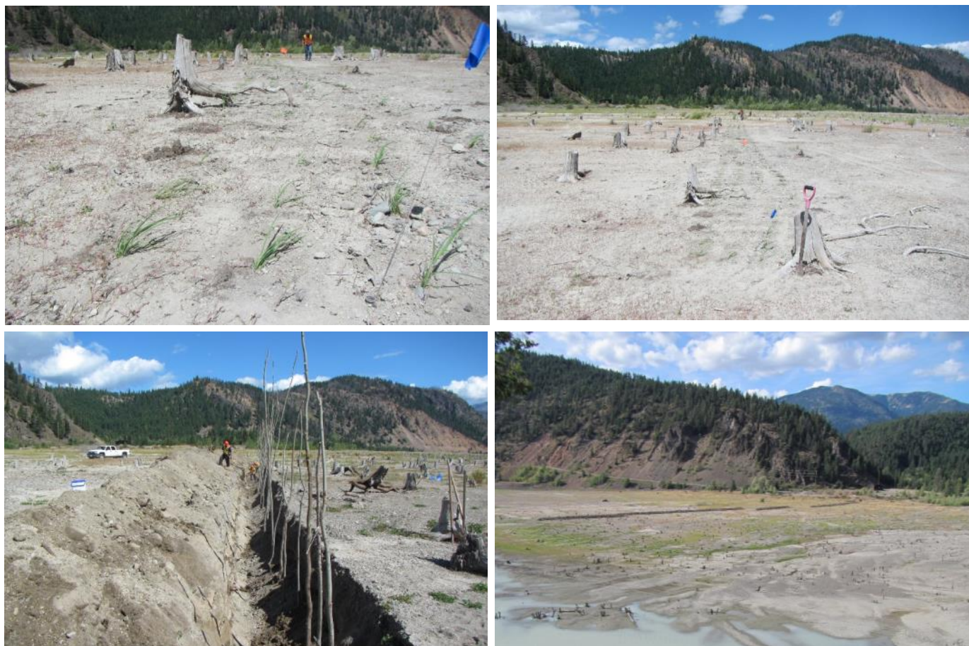
Figure 30 Gun Creek Fan west sedge strip planting and live stake cuttings trenches. Lower right photo taken from Truax FSR as machine was backfilling planted trenches.
