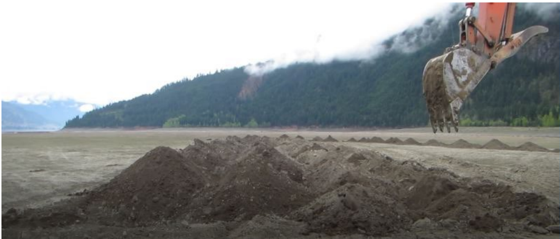
Figure 8 Mounding in 2017 outer mounds created with clean up bucket and inner with smaller digging bucket.
