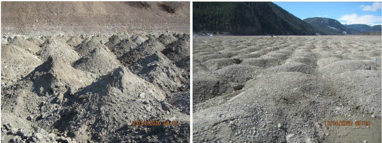
Figure 28 Examples of mounding treatment immediately post treatment on the left (MW1900A), and one year post inundation on the right (MW1900B).
