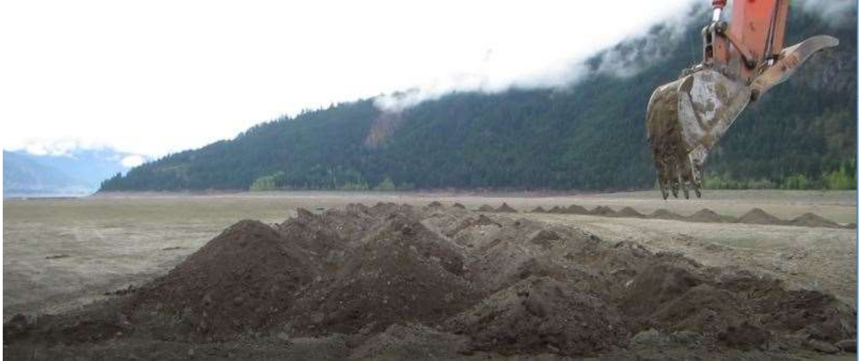
Figure 8. Two left hand rows of mounds done with clean-up bucket, right side done with toothed clean up bucket.
