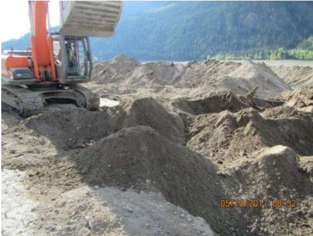
Figure 7. Polygon MW1702 being constructed using an excavator fitted with large volume clean-up bucket.
