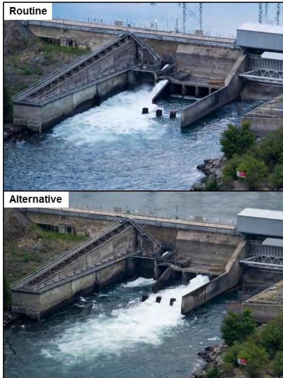
**Figure 3-8: Flow fields in the Seton Dam tailrace during routine BC Hydro operations of flow scenario 3 (top) and an alternative flow scenario (bottom)**
