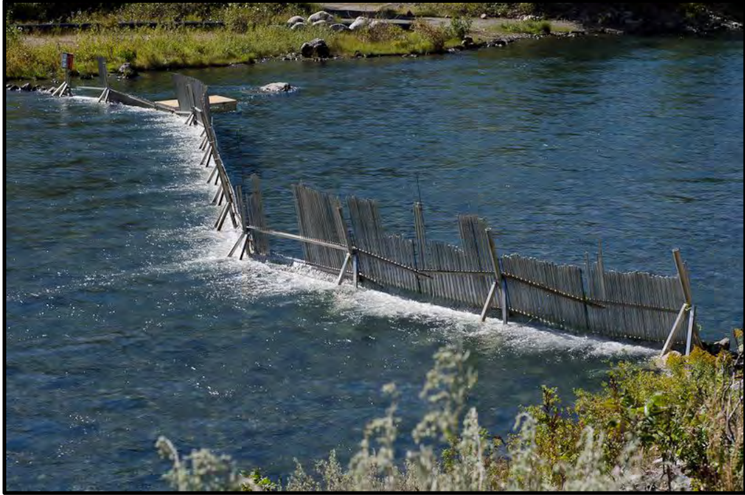
Figure 2-5: Full-spanning fish fence in the Seton River. Note open panels mid- and left-channel to allow upstream fish migration
