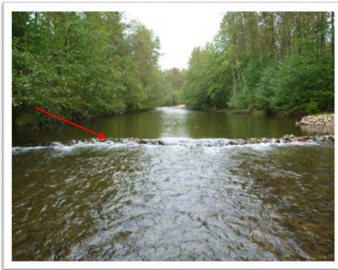
Figure 10 - Index site 2a - upstream view of weir, Sept.13.11 Discharge = 3.36cms (WSC Port Coquitlam) The arrow identifies the constructed weir
