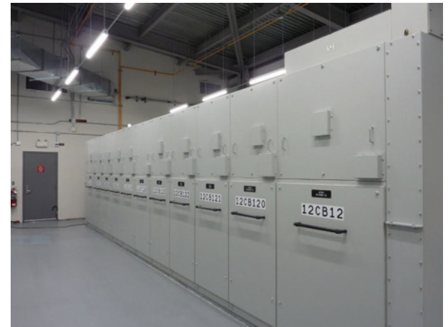
Capilano Substation Dry-air medium-voltage switchgear system
