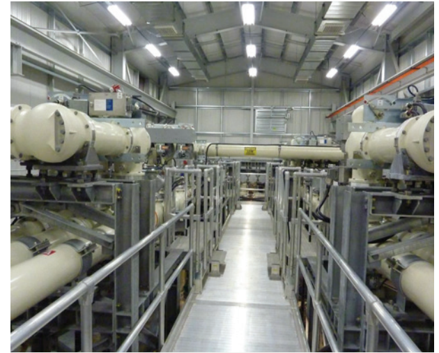
A 230 kV Gas Insulated Switchgear (GIS) Unit in Horsey Substation
