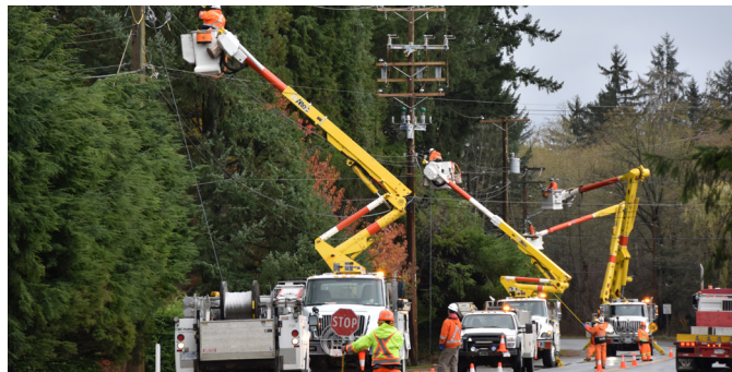
Campbell River crews installing reclosers along Highway 28.
