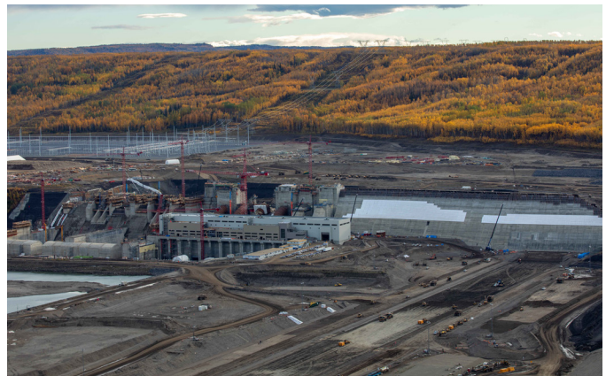
A view of the Site C dam core trench, dam buttress, powerhouse, spillways, and the operational substation in the background.
