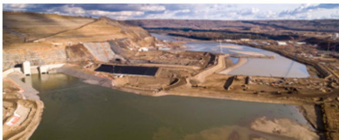
The Site C project achieved river diversion in October 2020.
