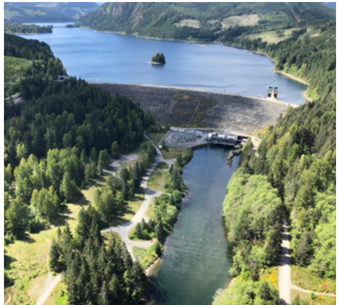
Strathcona Dam, one of the dams in the Campbell River system, is the largest dam on Vancouver Island.
