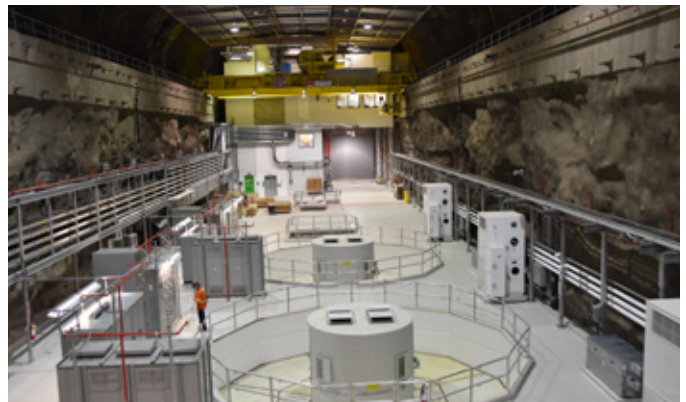
The underground John Hart Generating Station. The generating station's capacity increased by about 10% over the old facility, using the same amount of water. It creates enough power to serve about 80,000 homes.
