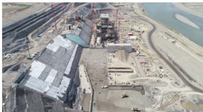
The Site C spillways excavation (foreground), powerhouse and main service bay, looking upstream, in July 2019.
