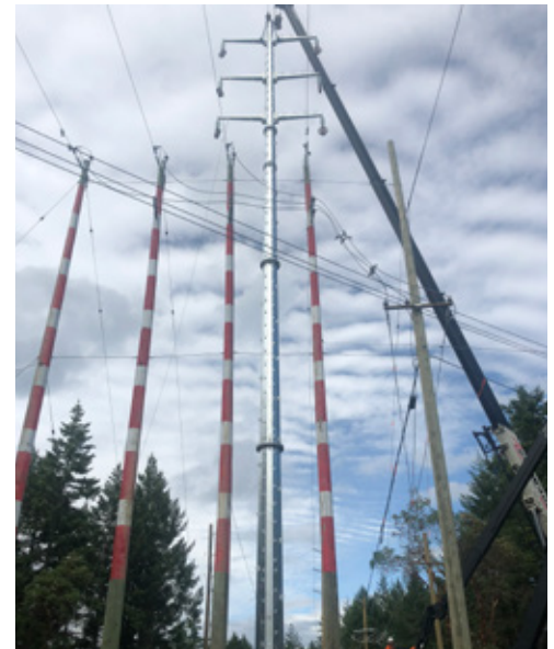
Mudge Island 2019 – old and new. The newly raised steel monopole in close proximity to the four pole wooden structures.
