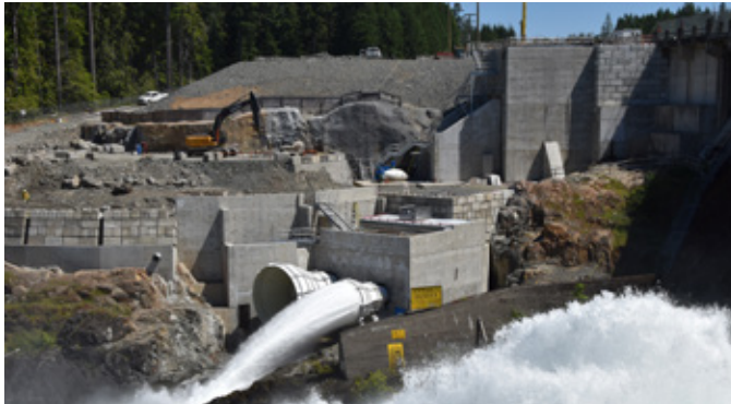
The water intake structure and low level outlet valves on the downstream side of the John Hart Dam. The intake goes under the dam with water passing into the power tunnel for power generation or to the two low level outlet valves.
