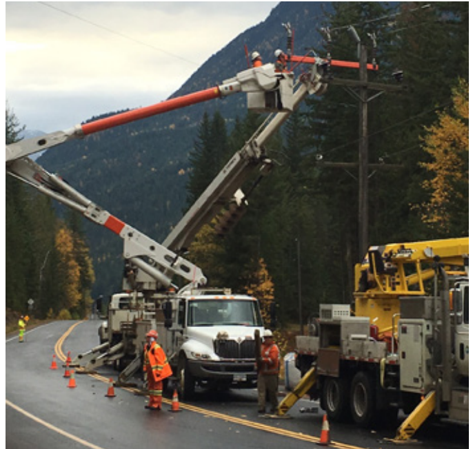
Crews use a special boom to safely lift the energized line and allow a new pole to be installed without turning off the power.
