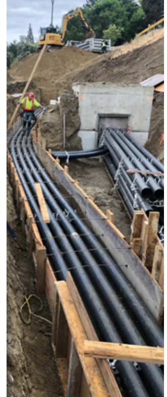
Undergrounding power lines in downtown Kamloops.
