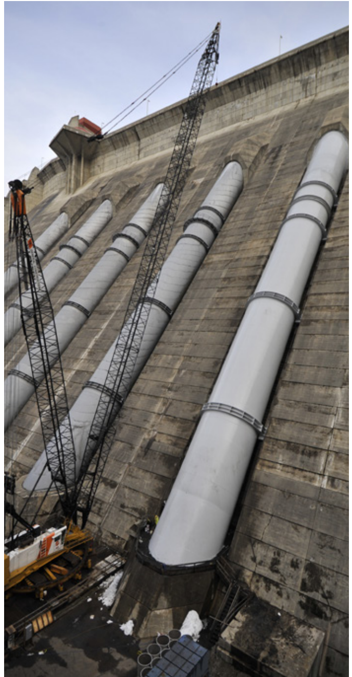
Installing the Revelstoke 5 penstock on the face of Revelstoke Dam.
