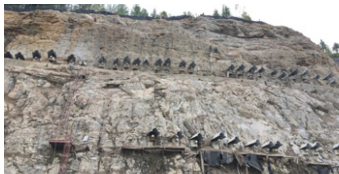
Installing protection for anchors.
