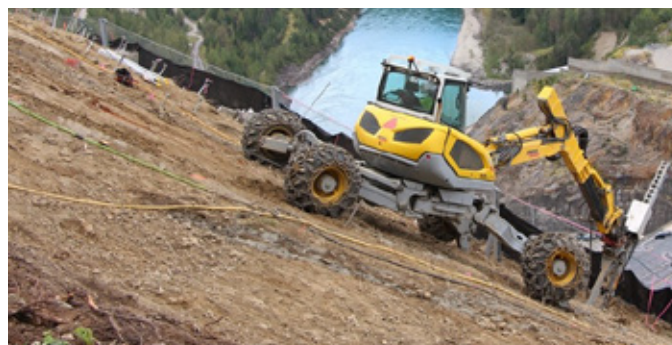
Tethered cat installing anchors.
