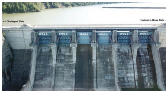
Peace Canyon spillway operating gates.
