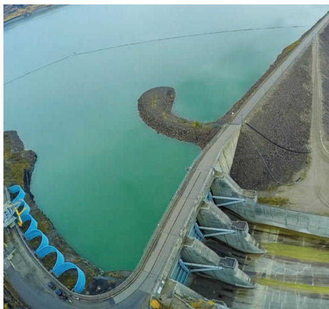
W.A.C. Bennett Dam spillway and existing debris boom.
