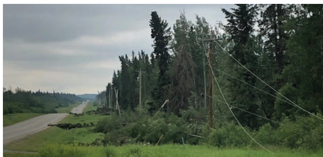
Downed lines from downburst winds: trees and power lines lay broken along Highway 97 north of Charlie Lake.
