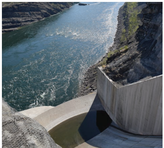
Flip bucket at W.A.C. Bennett Dam.
