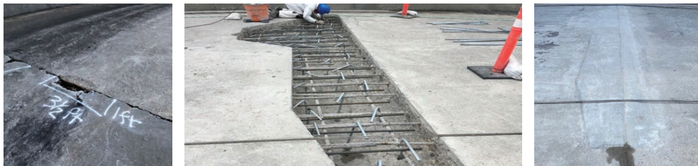
Before, during and after conditions of one remediated joint in the spillway.
