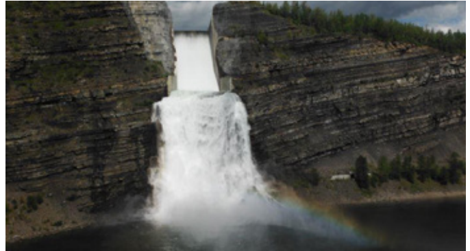
Water being released down the spillway during our testing of the spillway reliability upgrade work at W.A.C. Bennett Dam in summer 2019. Photo courtesy of John Verney, BC Hydro.
