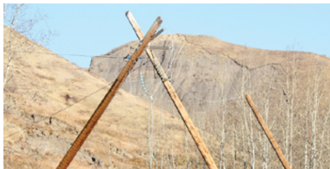
Power lines damaged after the Old Fort landslide. Photo courtesy of Matt Preprost of the Alaska Highway News.
