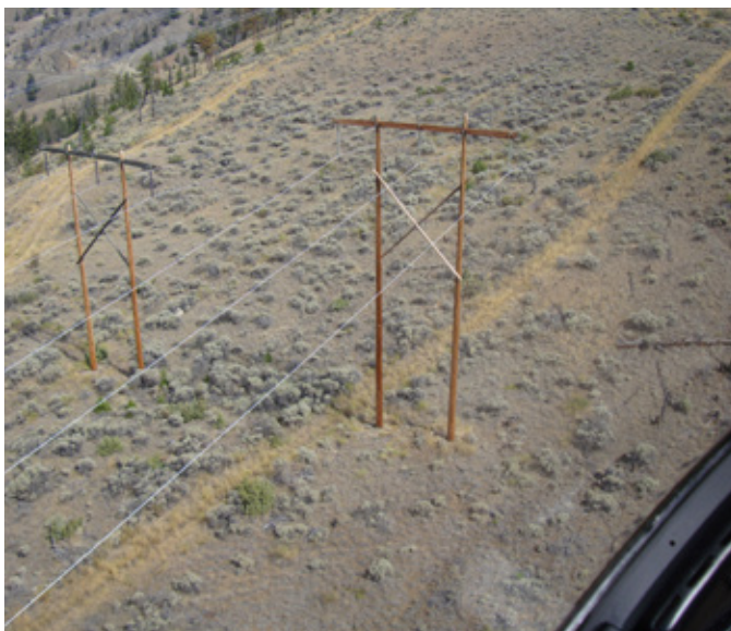
PRES will be a double-circuit 230 kilovolt line on parallel wood pole structures.
