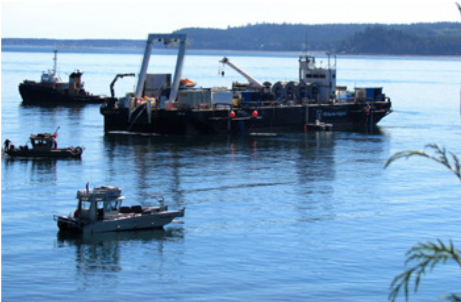
Cable pickup operation in progress using a dynamic positioning barge, divers, marine surveyors and a remotely operated undersea vehicle.
