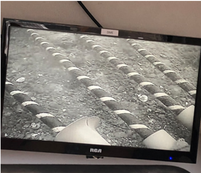
Diver’s cam shows three new cables on the sea bed while the fourth cable is being pulled through the duct.
