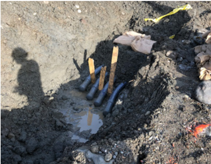
New cables will run in four new underground ducts placed from above high water mark to zero tide level at both ends of the crossing. This means no digging of beaches in the future and no cables exposed on the beaches.
