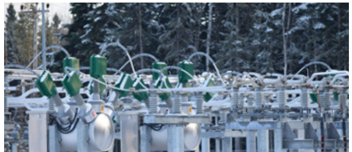
Animal mitigation equipment at Chief Lake Substation in Prince George.
