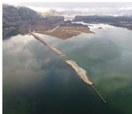
Nearly $350,000 of FWCP funding in 2021–2022 went to removing a section of berm in the Squamish Estuary in the Cheakamus River Watershed to improve fish passage. The Squamish River Watershed Society is leading the project and plans to remove more of the berm in 2023. Photo courtesy of: J. Buchanan
