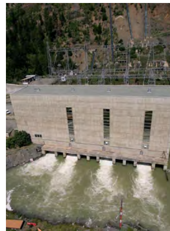
Bridge River 1 Generating Station in Shalalth
