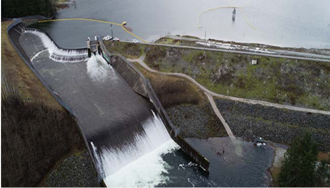
Aerial view of Alouette Dam and spillway.
