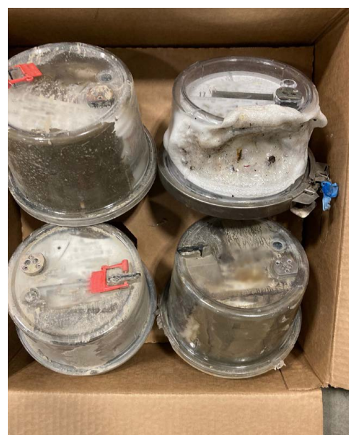
Damaged meters collected from properties in the Sumas area following the November 2021 floods.
