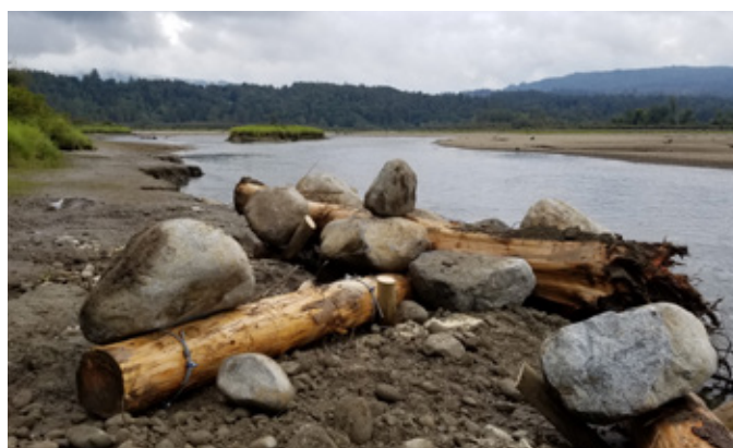
Floodplain restoration, using large wood and boulder structures, at Stave River. Photo credit: N. Cox.
