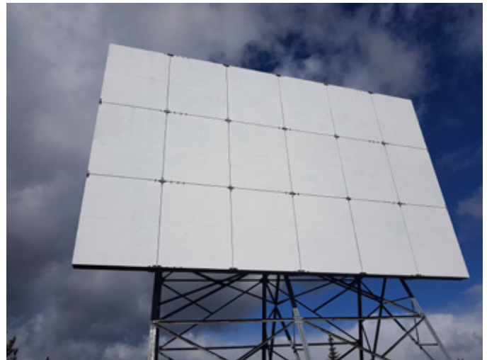
The updated passive reflector north of Sparwood. A passive reflector is a large reflective panel that helps to complete a microwave link when there are obstacles in the path. In this case, mountains block the direct path between Natal Substation in Sparwood and Morrissey Ridge, south of Fernie.
