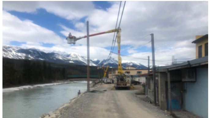
BC Hydro crews remove overhead infrastructure during the Golden dike improvement project in April 2020.
