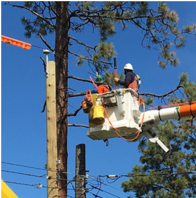
Powerline technicians work to swap out an end-of-life pole in Cranbrook in June 2020.
