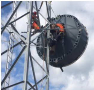
Crews work to install a microwave on the newly installed tower at Natal Substation.
