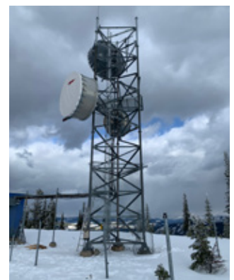
The microwave tower at Morrissey Ridge, south of Fernie, was extended in height by two metres.
