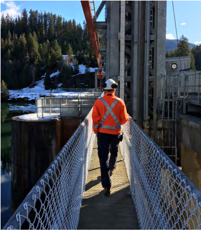
A walk down the Seven Mile Dam causeway. Photo by Megan Chadwick.
