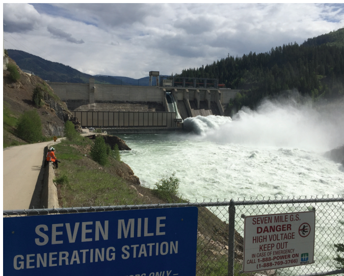
Seven Mile Dam and Generating Station. Photo by Martin Gedig.
