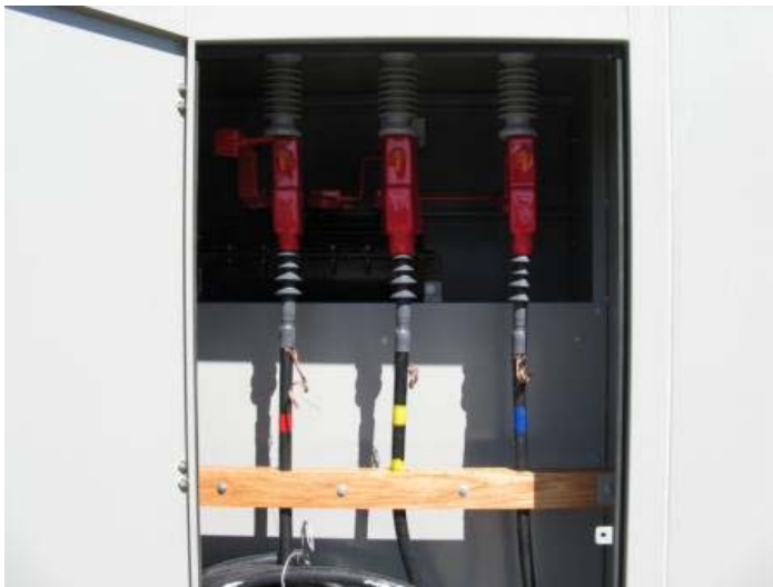
Primary cable compartment
