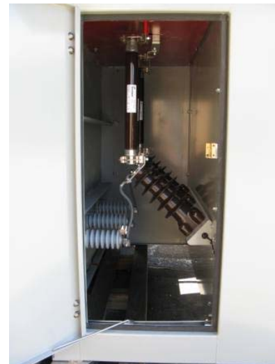
Customer-owned primary fuse compartment
