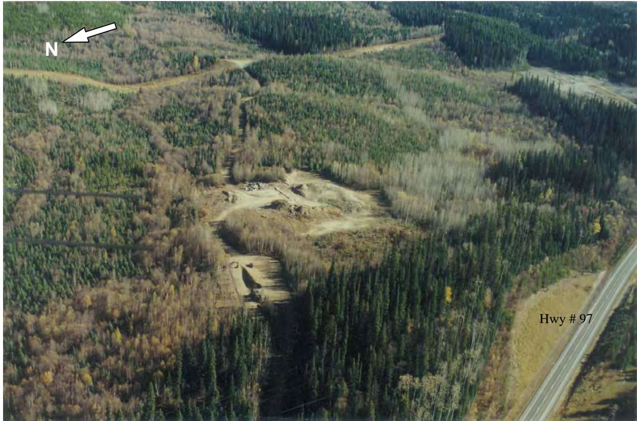
Figure 3. Aerial view of the McLeod Lake Landfill, looking southwest.
