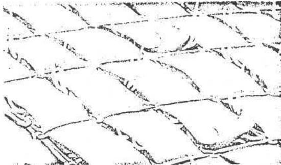
Figure 42 - Biodegradable Material Provides Soil Stabilization Until New Growth is Established (Anco Chemicals Ltd, Maple, Ontario)
