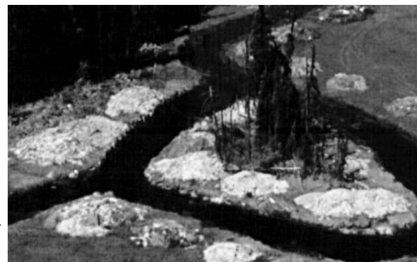
Level ditching channels created in marsh area at Neilson Lake.
