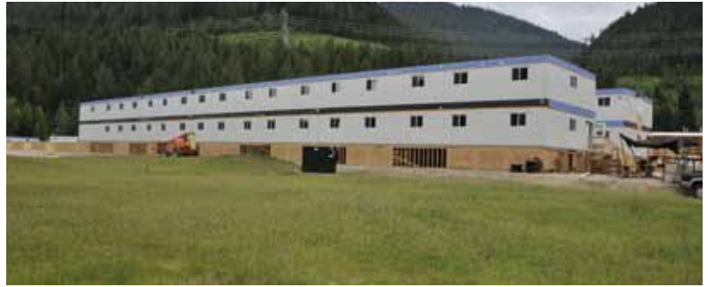
New single-room dormitory building for BC Hydro's expanded Mica Creek camp.
