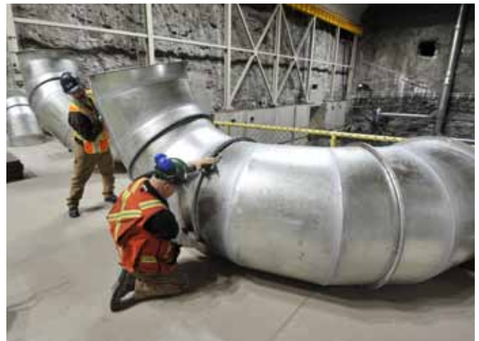
Crew assembles ventilation ducts.
