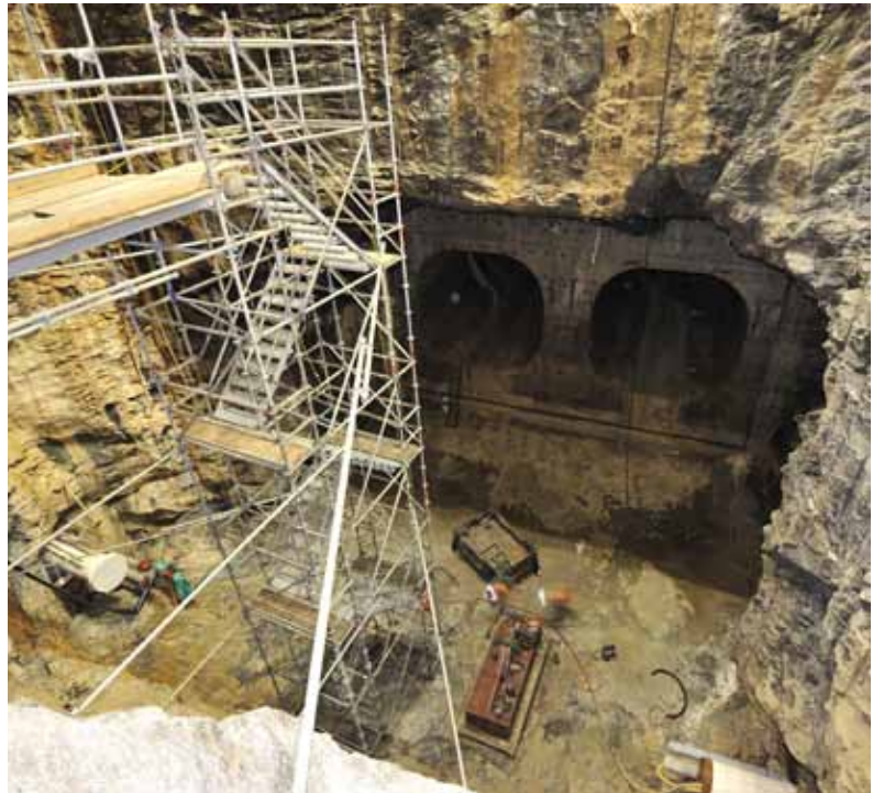
Draft tube for new fifth Mica generating unit.
