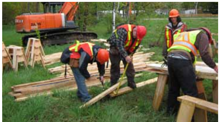
Okanagan College residential construction students receives hands on training at job site in Revelstoke.
