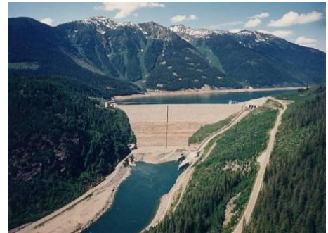
Earthfill dam at Mica Generating Station
