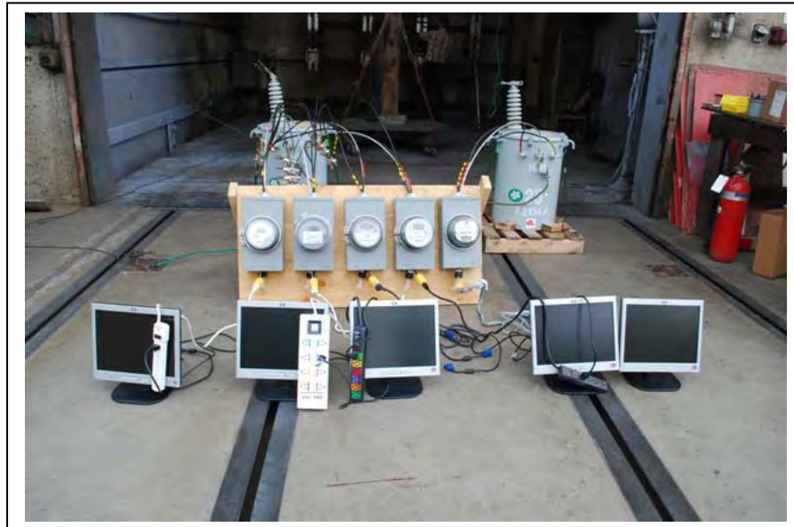
Figure 5 – Final Test Set-Up for Over-Voltage Tests
