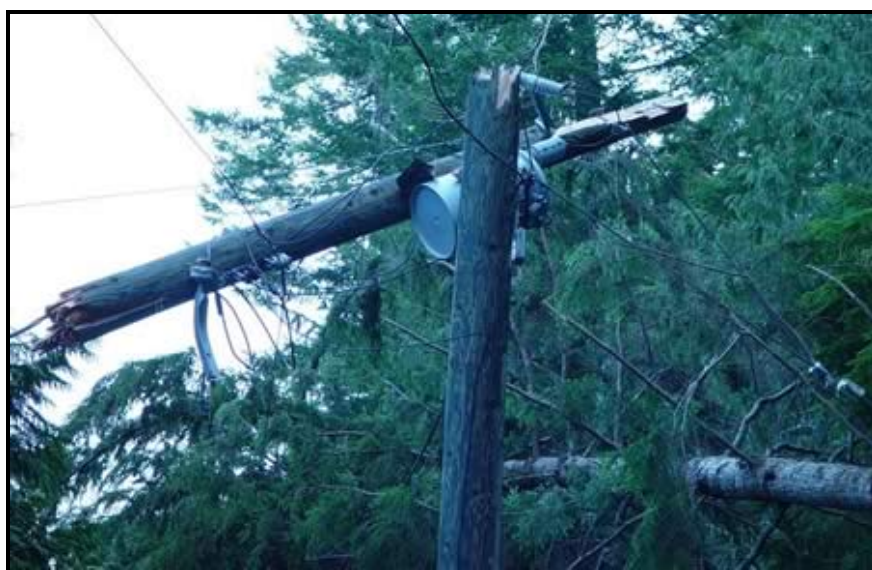
Trees and adverse weather are the most significant causes of outages, totaling 77% of all customer-hours lost for fiscal year 2007.
