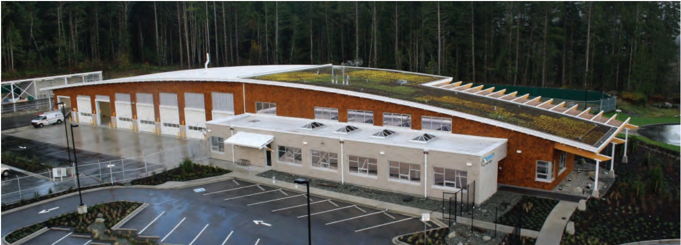
In operation since 2010, the new Port Alberni office building has been designed to meet current and future operating requirements and provincial energy building standards. The building’s features include a geoechange heat pump system, solar hot water heating panels and a vegetated roof.
