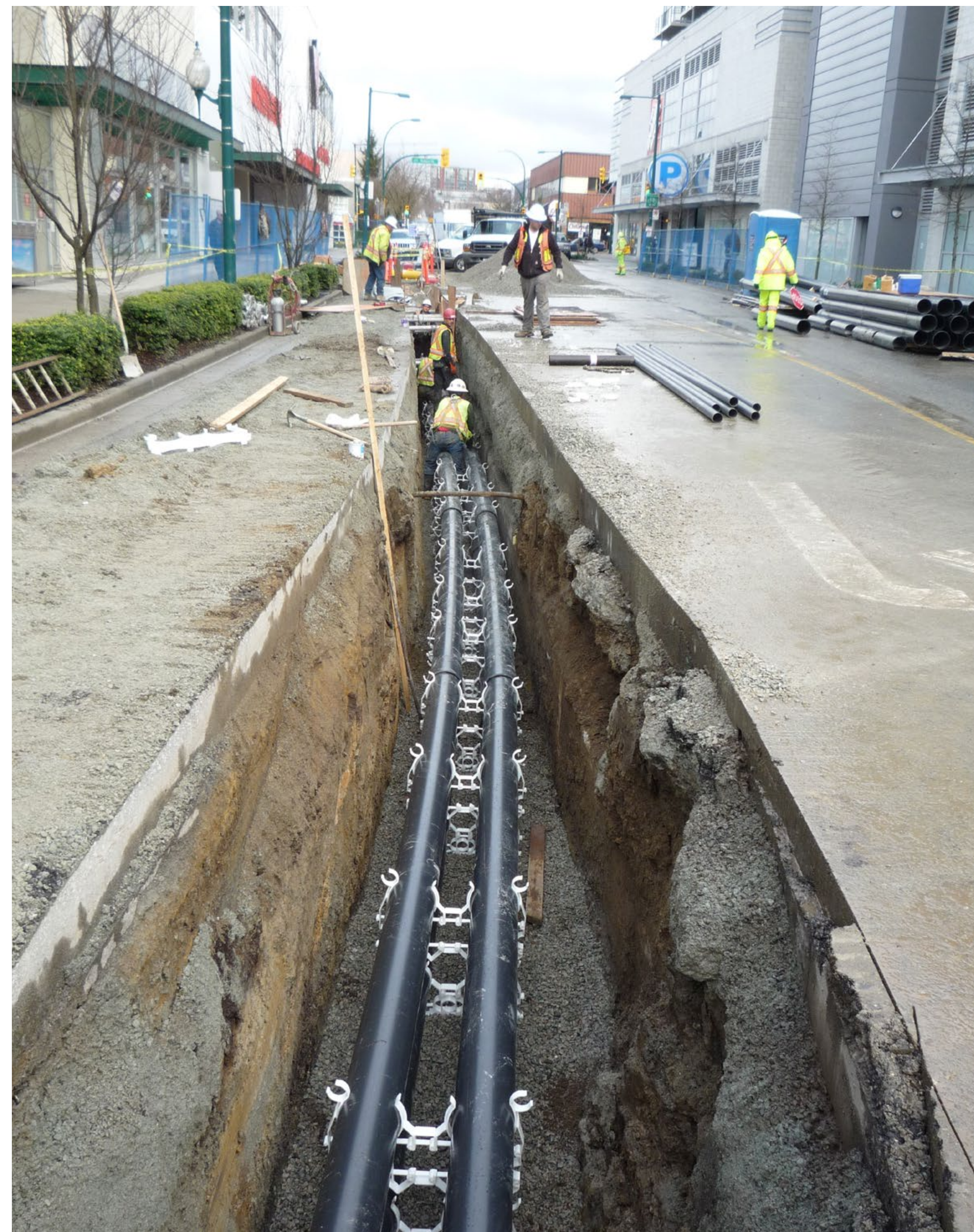
Typical underground cable duct bank installation
