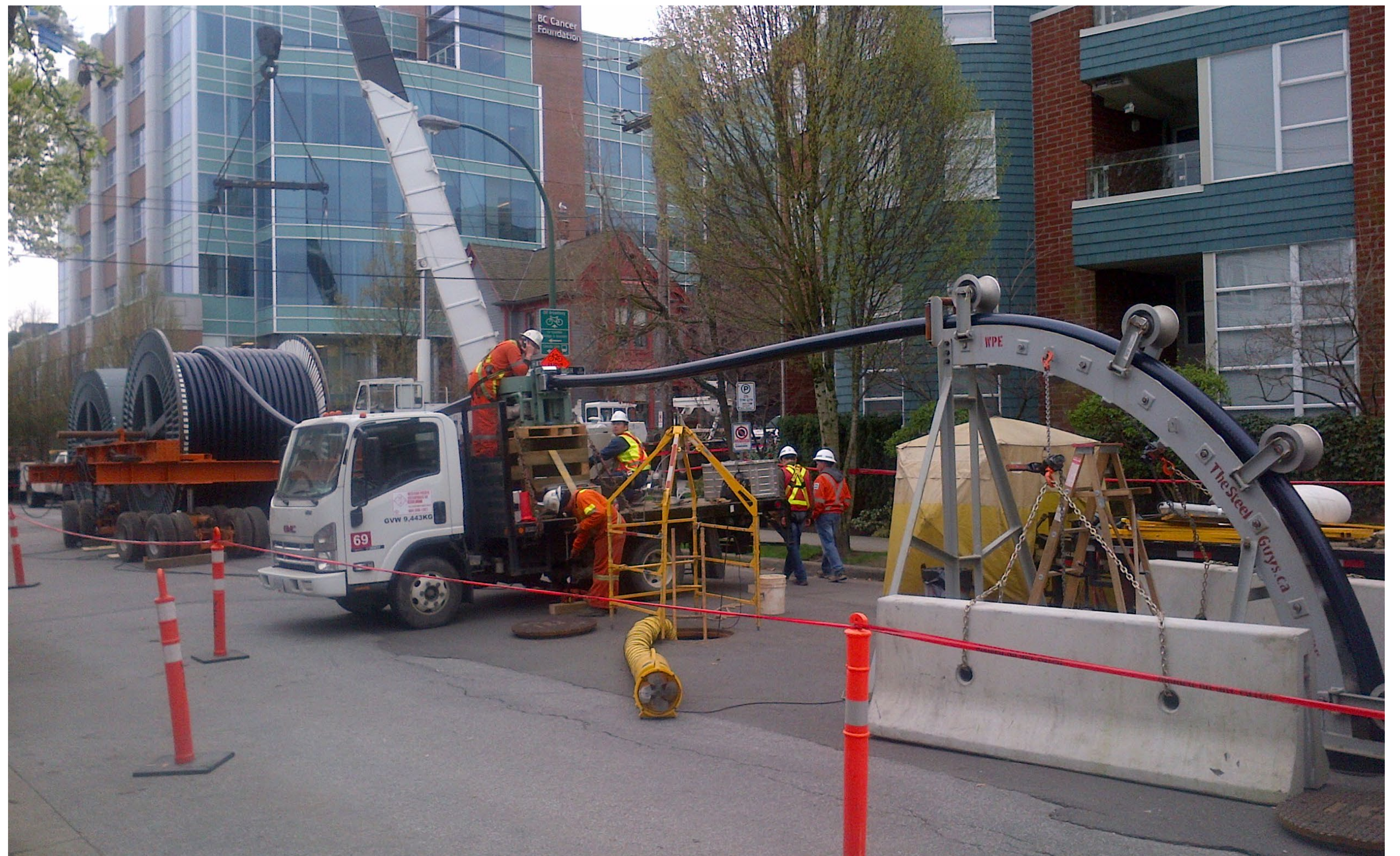
Typical underground cable pull
