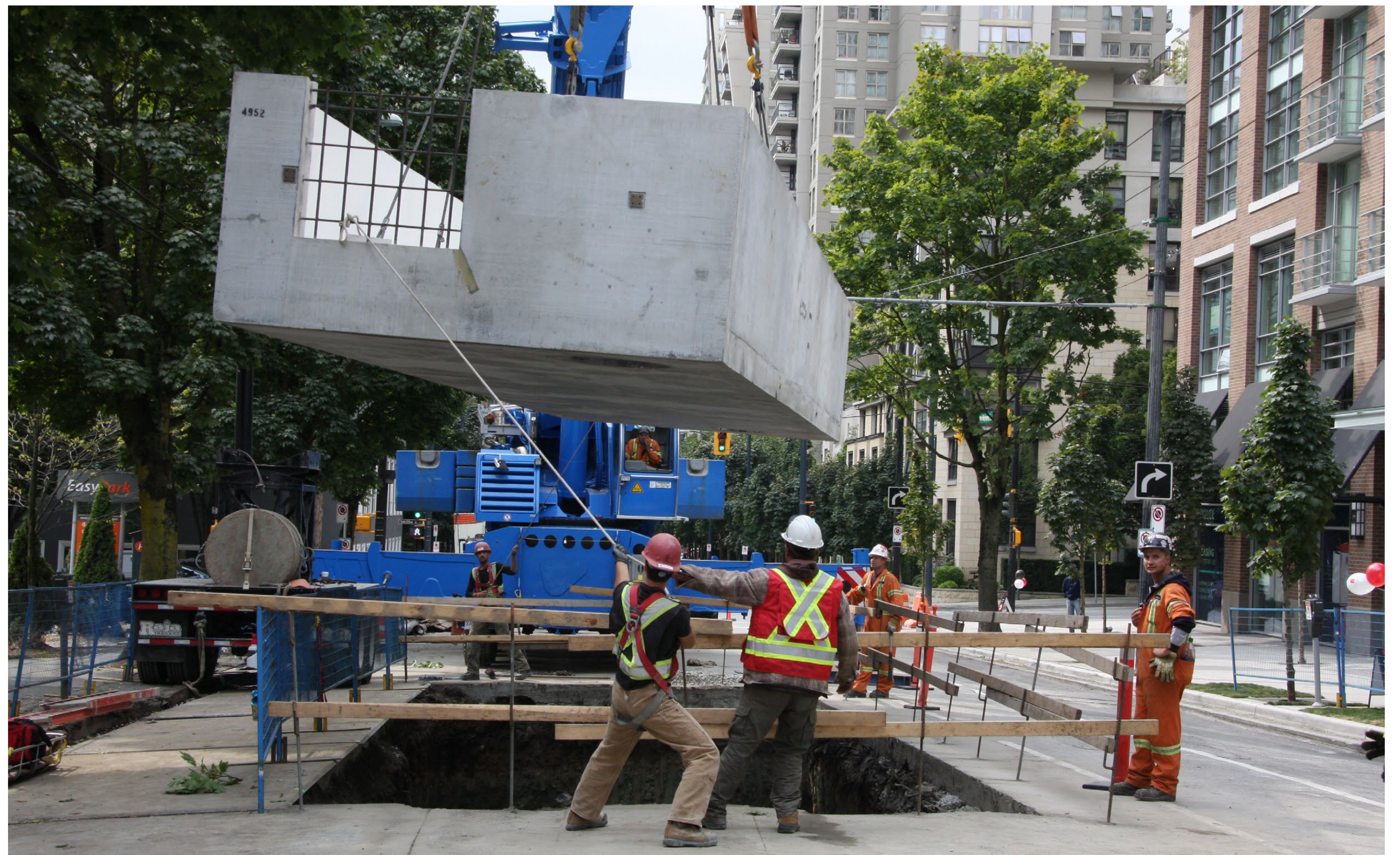
Typical manhole installation
