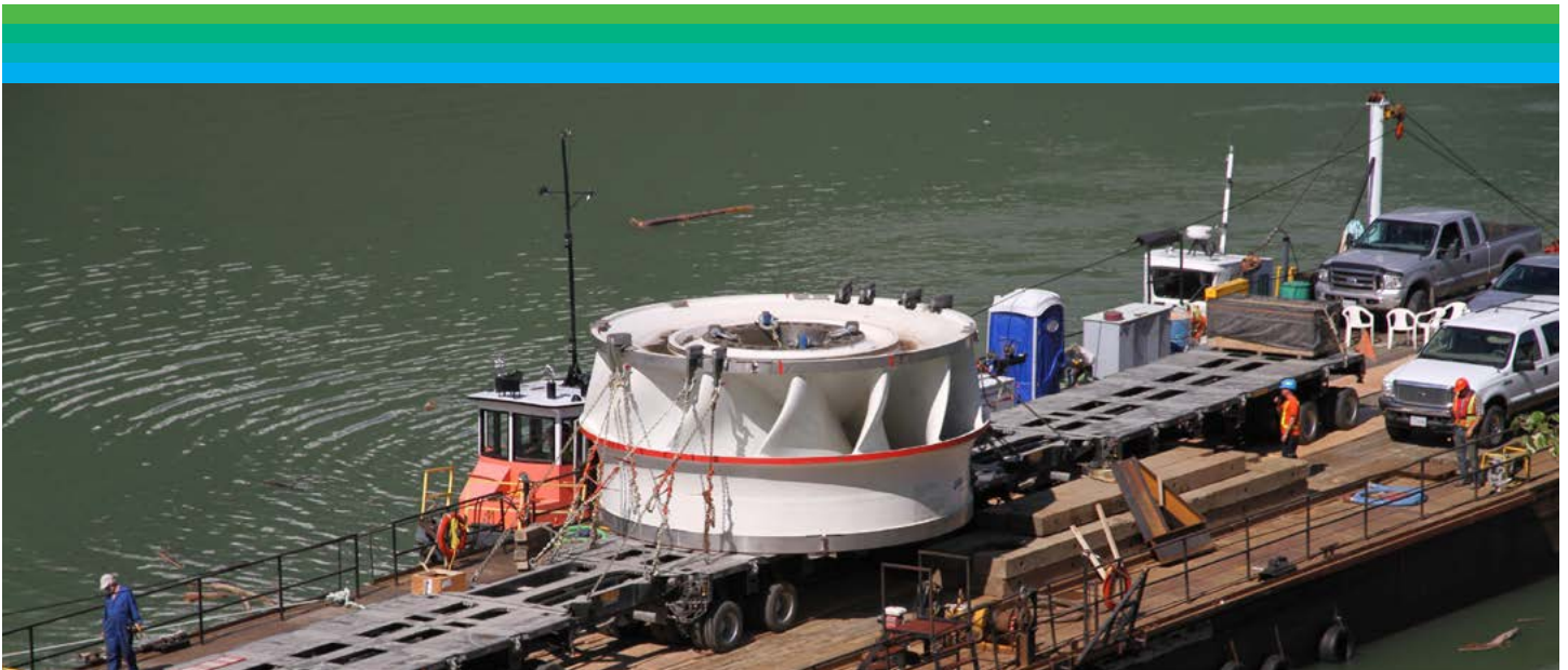
Barge transport of new turbine down Kinbasket Reservoir to Mica dam
