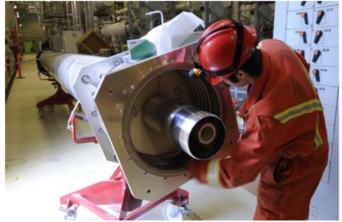
Inspecting gas-insulated switchgear
