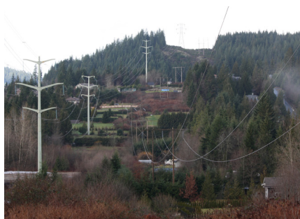
This right-of-way through the Village of Anmore was established in the 1960's.
