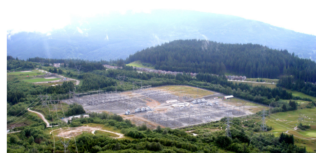
Alternative 2 would run from the Meridian Substation (pictured), in Coquitlam, to the Mount Pleasant Substation in Vancouver.
