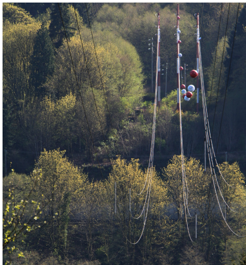
Existing Burrard Inlet crossing, looking south
