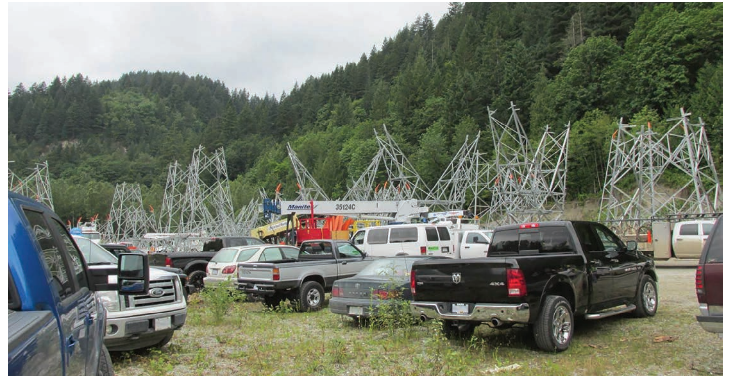
Crews assembled tower parts on the ground in one of the project's fly yards. Helicopters picked the parts up and flew them to site.
