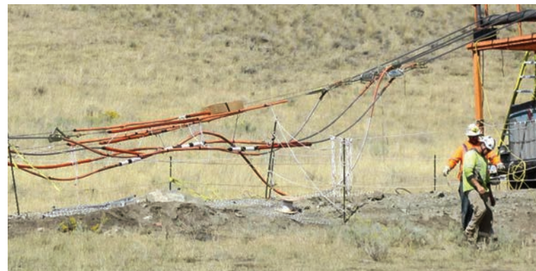
View of conductors and implosive sleeves prior to implosion.
