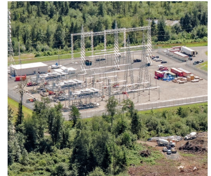
View of the Ruby Creek Capacitor Station.
