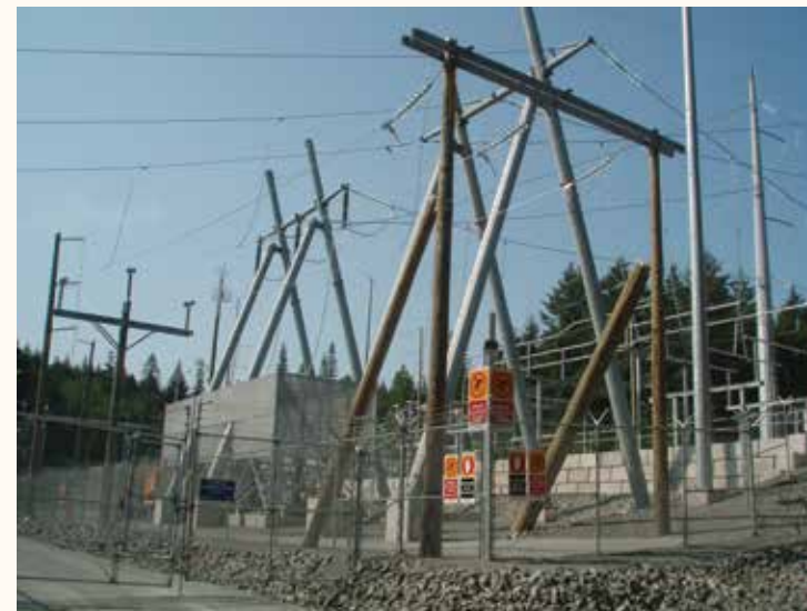
BC Hydro pothead at English Bluff, Tsawwassen. Potheads for this relocation would likely be similar in appearance to this pothead.
