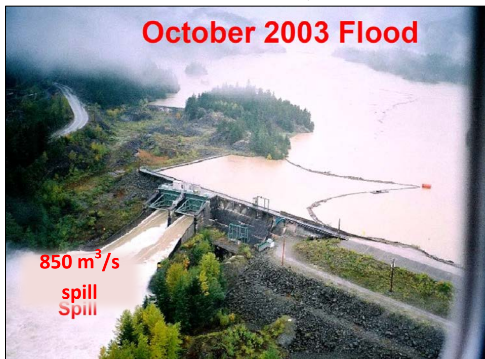
Spilling in October 2003 from Cheakamus Dam
