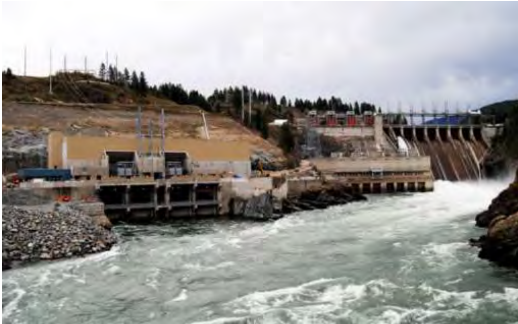
Figure 2-1 Waneta and Waneta Expansion
