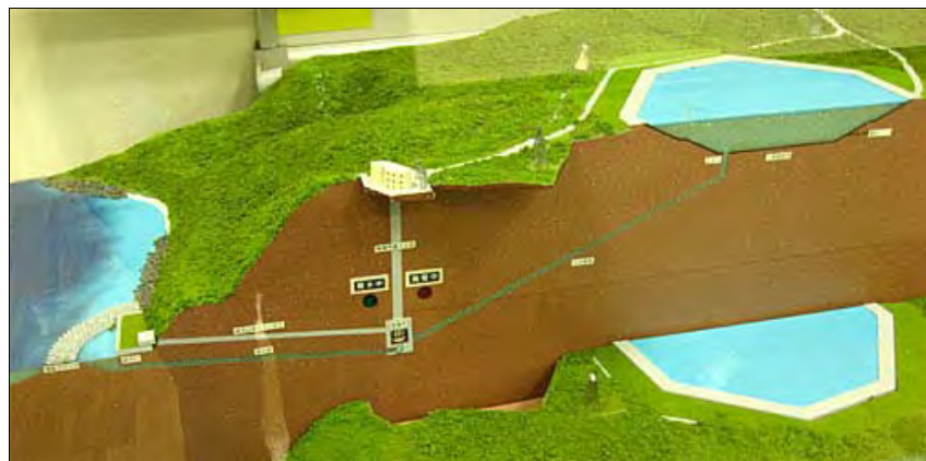
PHOTO 6 – Okinawa Saltwater Pumped Storage Plant – Cutaway Model of Plant.
