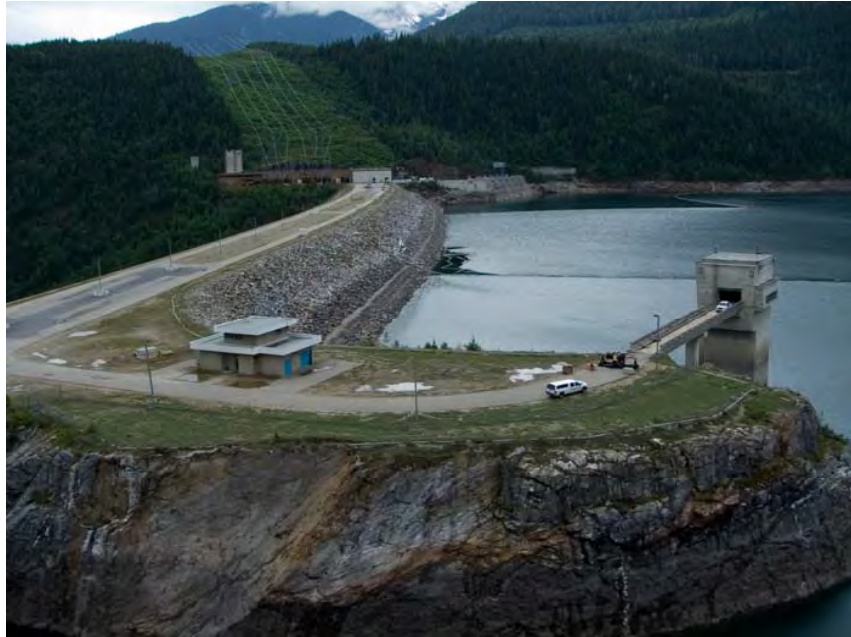
Photo 1 Mica Dam Crest showing Outlet Works Structure Beaker Building and Trans Lines
