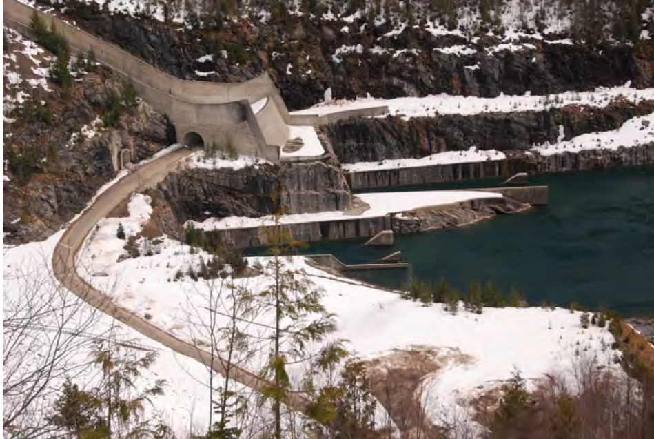
Photo 3 Mica Dam Left Bank Discharge Chute and Access Tunnel Portal to Diversion Tunnels
