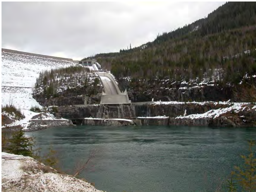
Photo 2 Mica Dam Left Bank, Outlet Works Discharge Chute and Spillway
