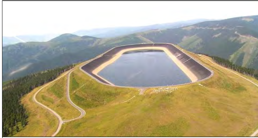
PHOTO 13 – Example of “Crow’s Nest” Upper Reservoir – Dlouhé Stráně Facility, Czech Republic.
