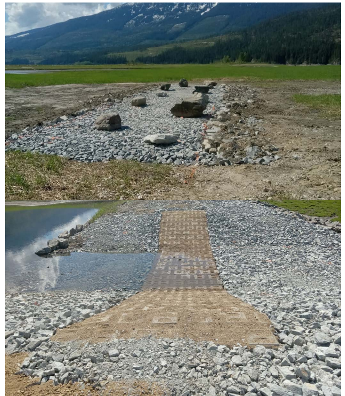
Completed remediation work at Cartier Bay, May 2023
