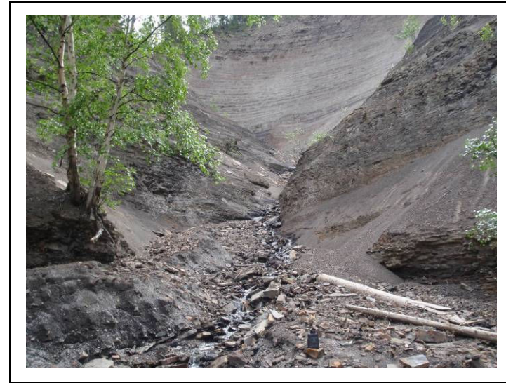
Plate 2. View of the gradient barrier on unnamed creek (230-803000), 96 m upstream from the reservoir confluence.
