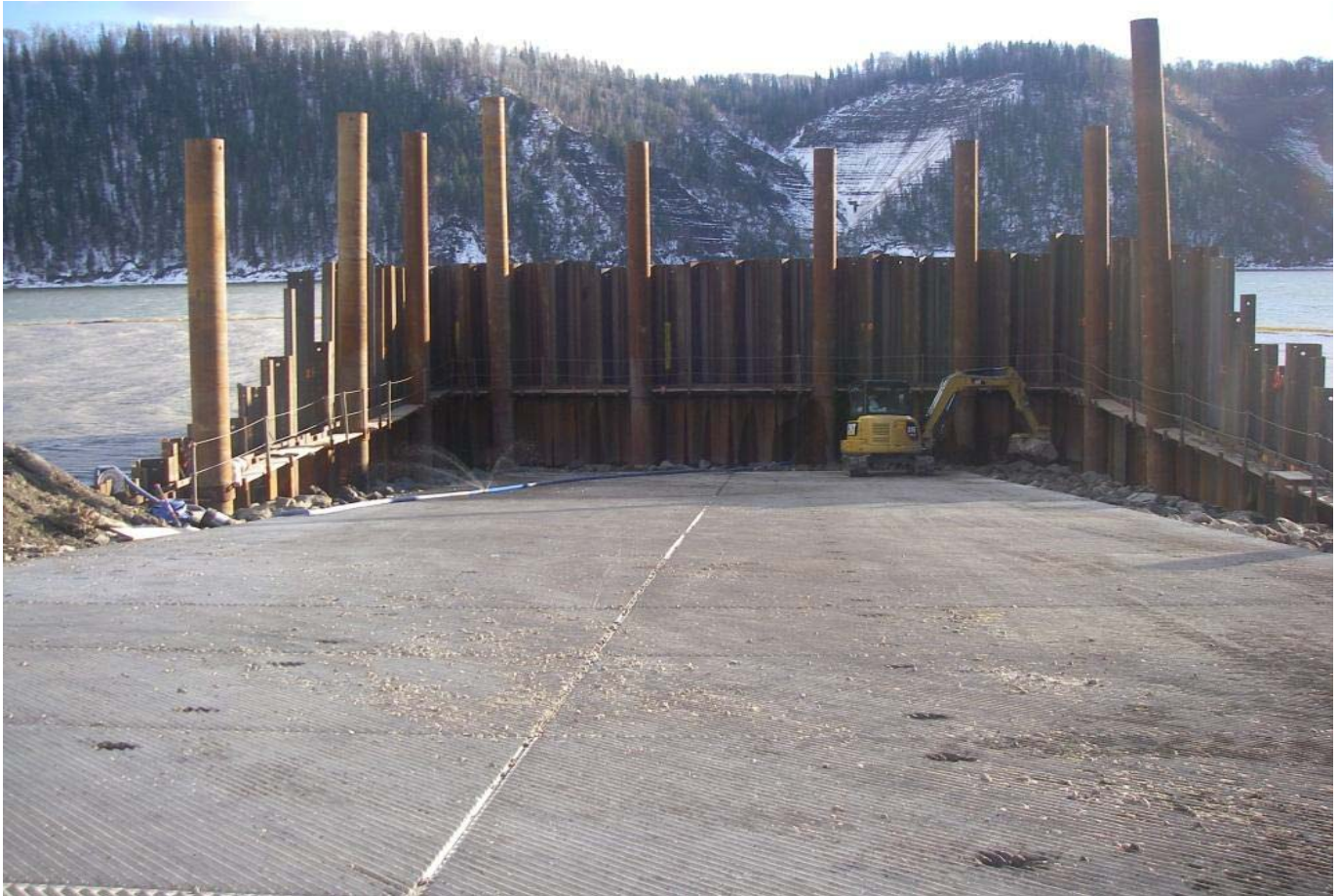
View of double lane ramp behind coffer dam during construction
