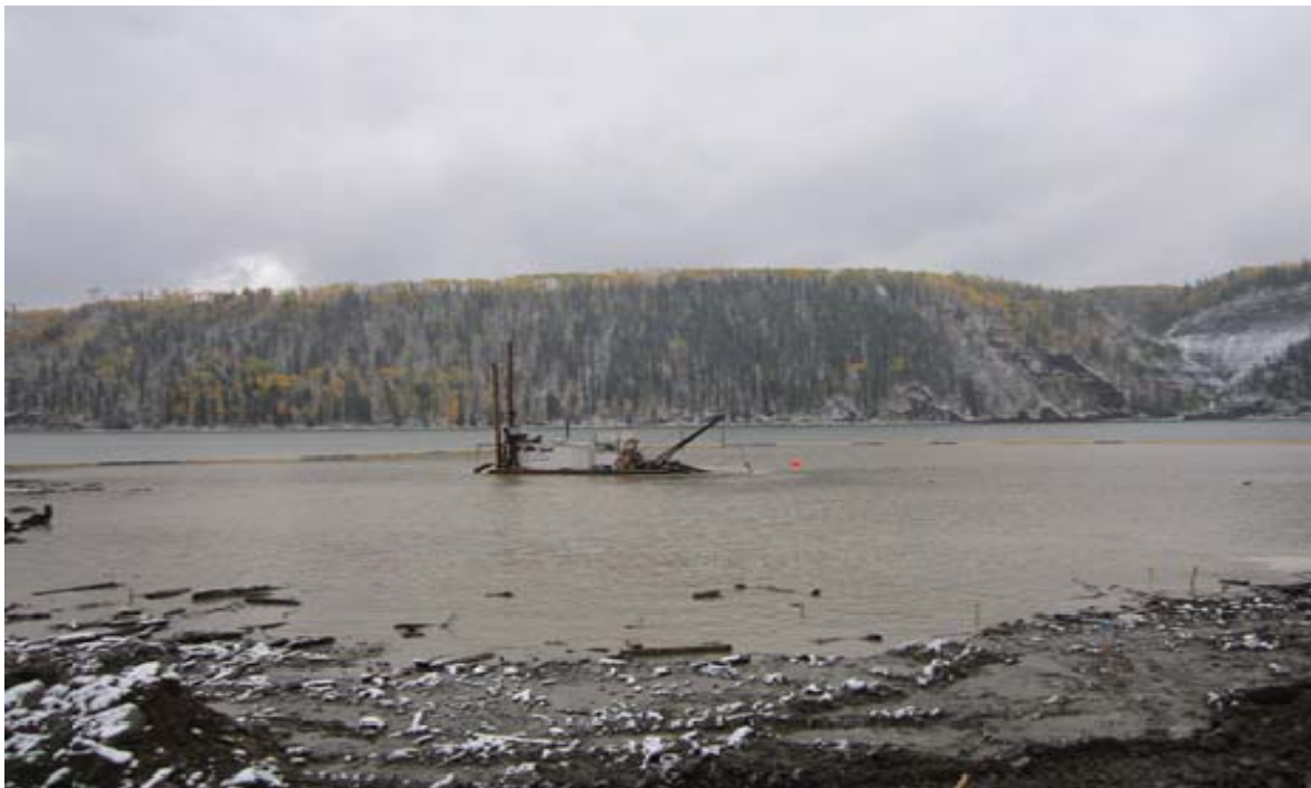
Dredging the boat basin
