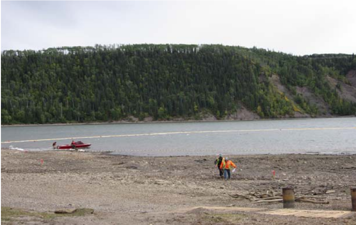
Turbidity curtain install around site
