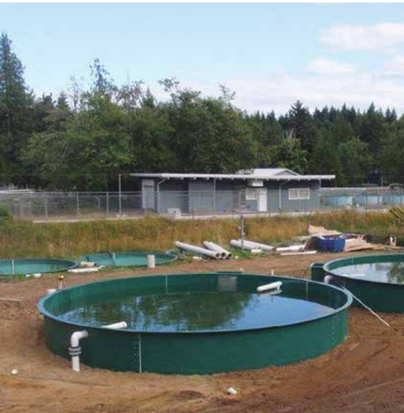
Photos: Open and shaded tanks improve salmon productivity at Qualicum Hatchery
