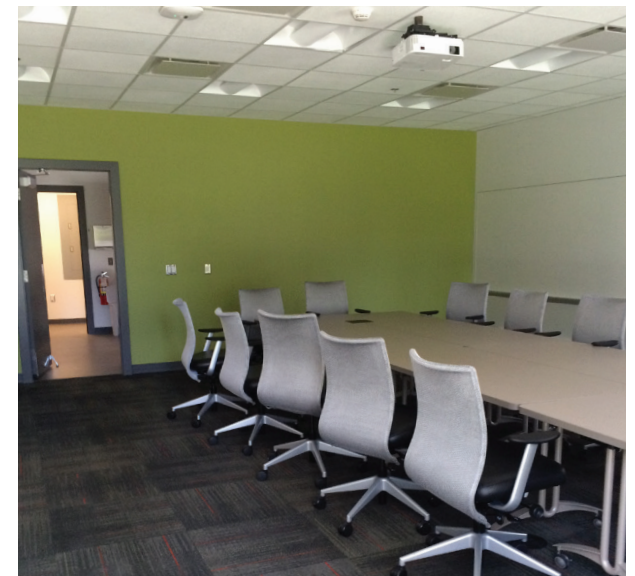
Interior lighting, Heating, Ventilation and Air Conditioning and direct digital control upgrades.
