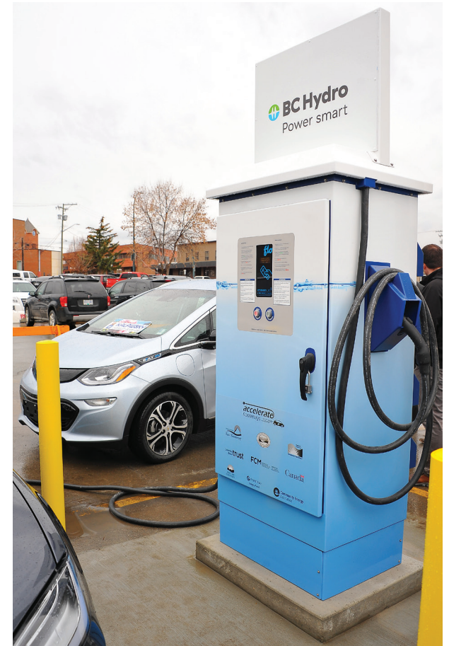
Fast charging station in the Columbia Valley.
