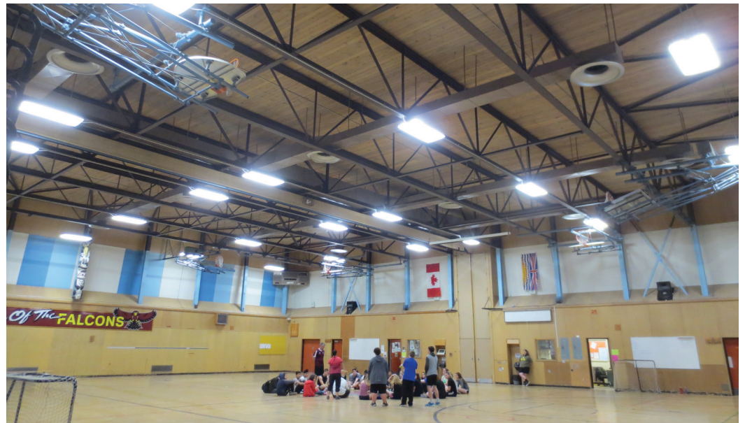
Lighting system retrofit at Lake City Secondary school.
