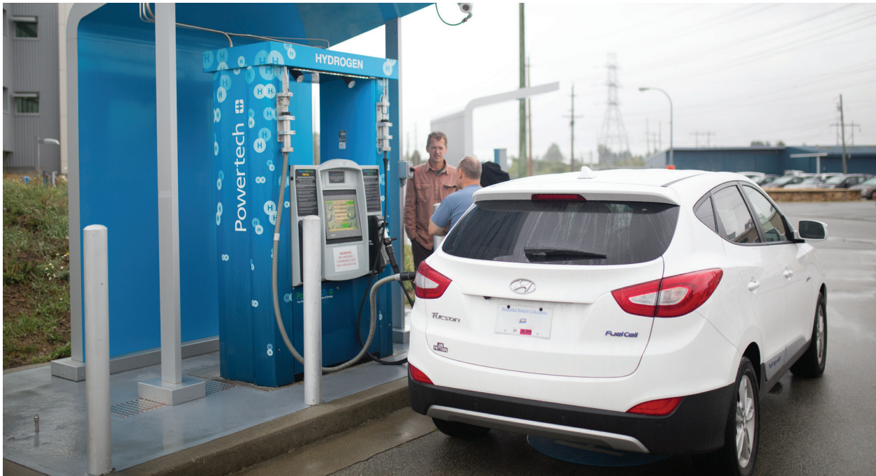
Powertech Fast-fill hydrogen fuelling station.
