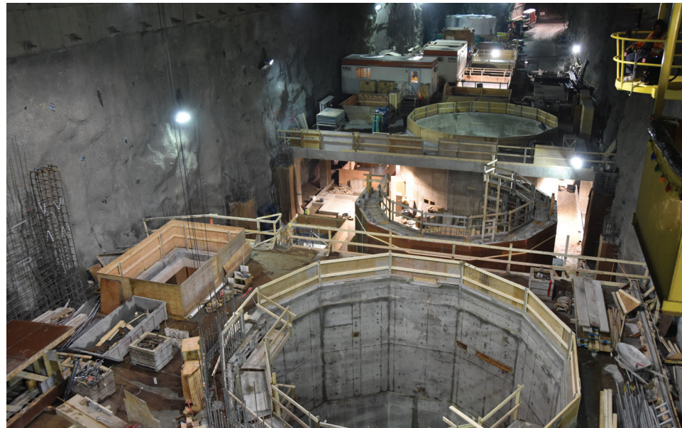
John Hart GS turbines under construction.
