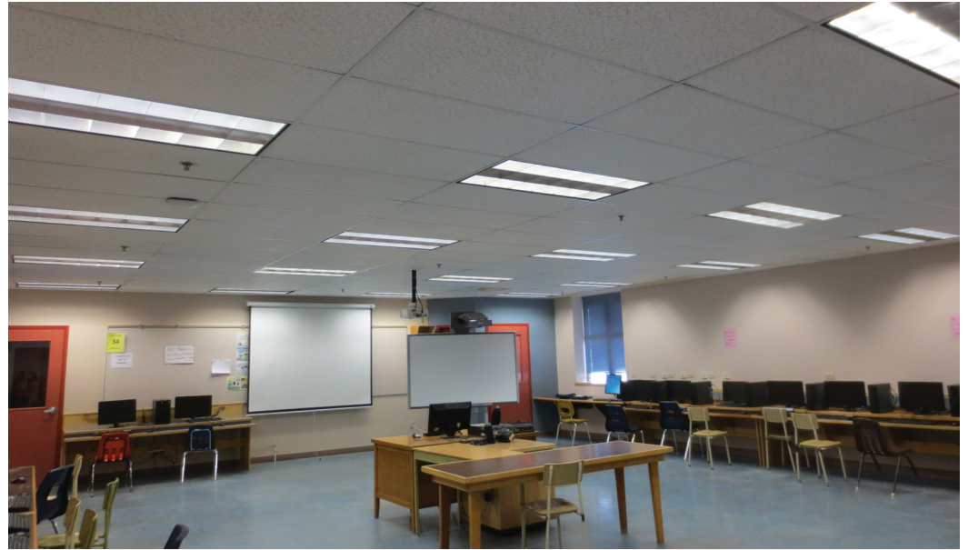
Lighting system retrofit in Lake City Secondary classroom.
