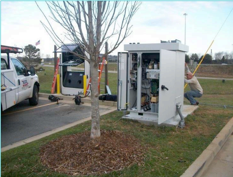
Figure 11-5 DCFC Installation
