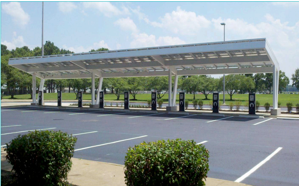
Figure 7-2 Level 2 Public Charging Station with Shelter and Lighting
