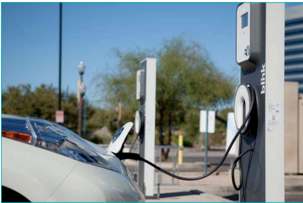
Figure 1 Nissan Leaf charging at AC Level 2 EVSE
